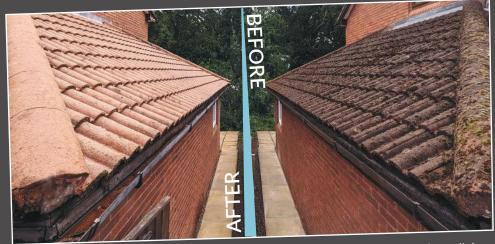
The process is carried out by washing the building from roof top to floor, and catching all the moss, dirt and lichen onto waterproof sheets, before simply disposing of the waste. Check out the video that covers the whole process, to see how this new method is not only safe and effective, but the perfect cost effective solution for carrying out roof cleaning with ultra impressive results.
